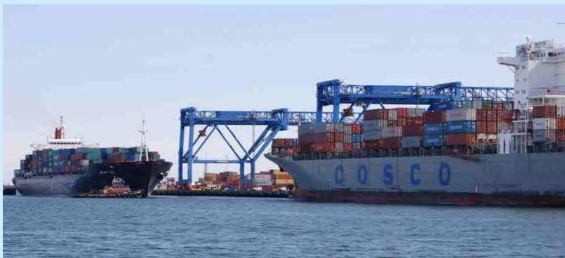
Conley Container Terminal
