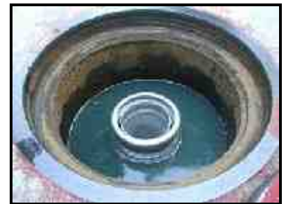
Spill bucket that contains liquid
