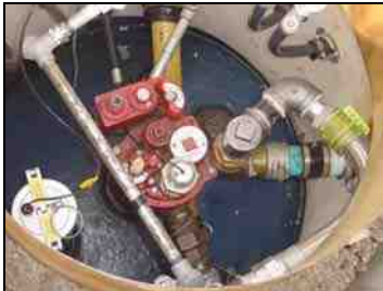
Contained turbine sumps and equipment in good condition
