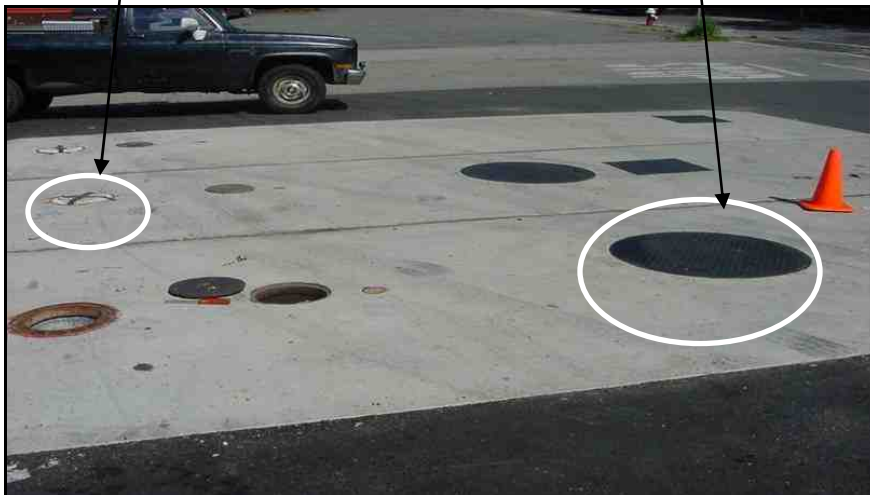
View of sump lids
