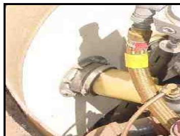
Sump penetration seals in good condition
