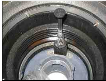
Spill bucket drain valve
